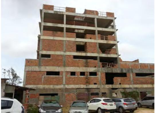
A photograph showing the north view of the building under construction. The structure is seen from a slightly lower angle, showing the brick walls and concrete framework. Several cars are parked in front of the building. |
